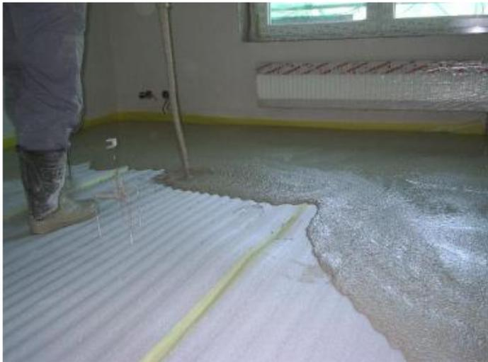
*Fast application of insulation on flat PBG subbase*
